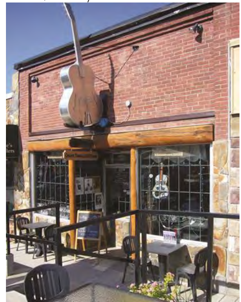
Figure 13 - Main Street business facade
