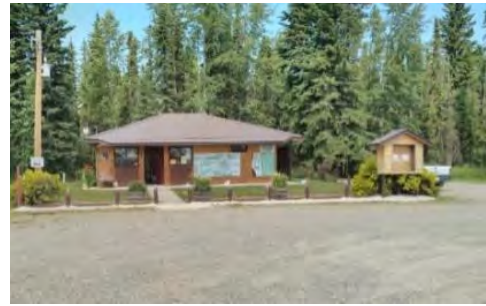
Figure 7 – Visitor Information Centre at Heritage Park
