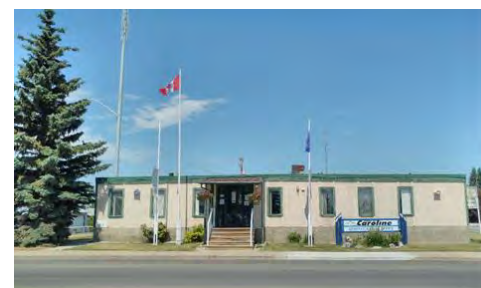
Figure 6 - The Village Office could benefit from signage and a façade update
