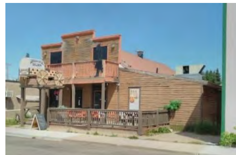
Figure 5 - Western Style facades found on buildings along 50th Ave
