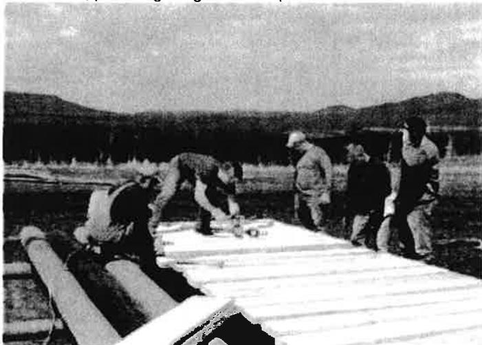
Volunteers, prefabricating bridges at Bill's place
