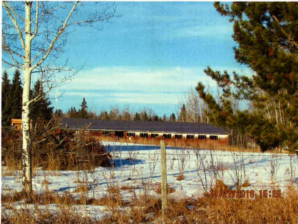
Barn/storage building (north portion of land) for proposed vehicle storage business
